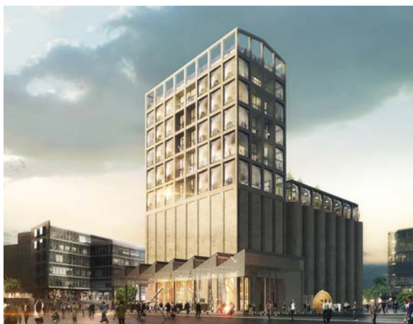
The Silo is being built in the grain elevator of the Grain Silo Complex
