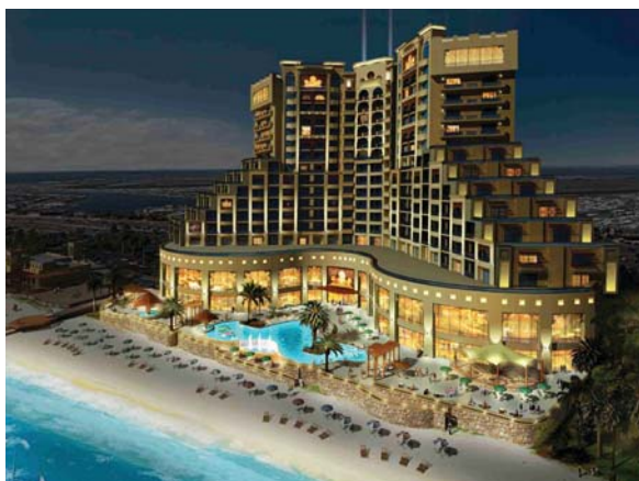
The 14-storey hotel houses 252 bedrooms and two-storey penthouses
