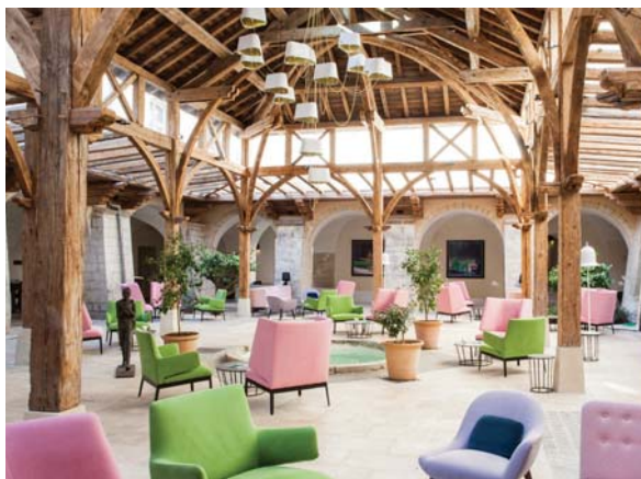
The courtyard timber structure is by Les Compagnons du Tour de France
