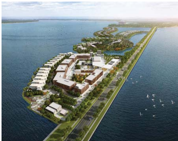
Sangha is being built along Yangcheng Lake outside of Suzhou
